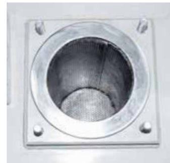
Installed inox filter.
